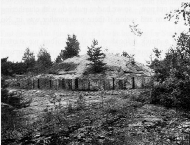
Vainode North R-14U/SS-5 base, concrete dome silo covers. Photo by Tim Robinson
